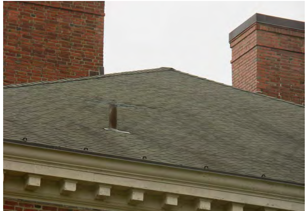
8. Spot roofing shingles missing
