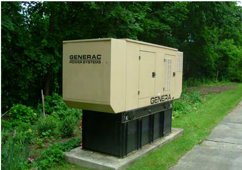
19. View of the emergency generator
