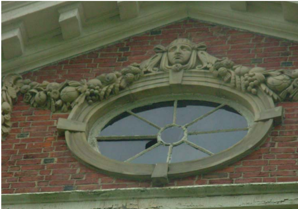
7. Original gable window to be repaired - re-built - replaced
