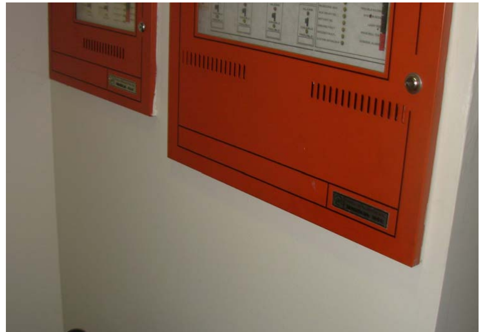
20. Main fire detection - monitoring panel
