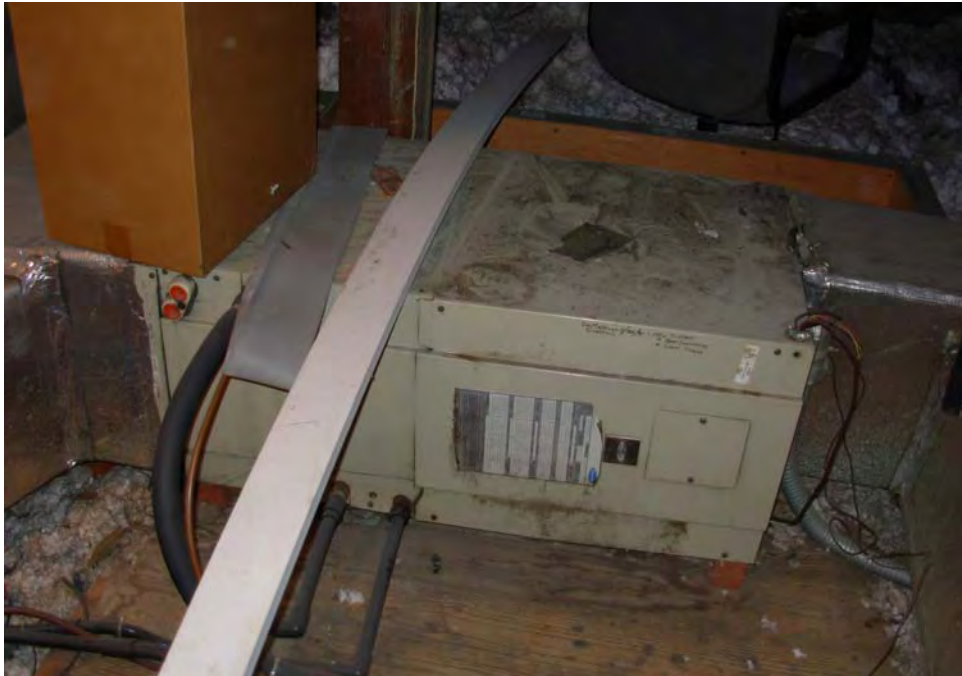
17. Community facilities' air handling unit in attic
