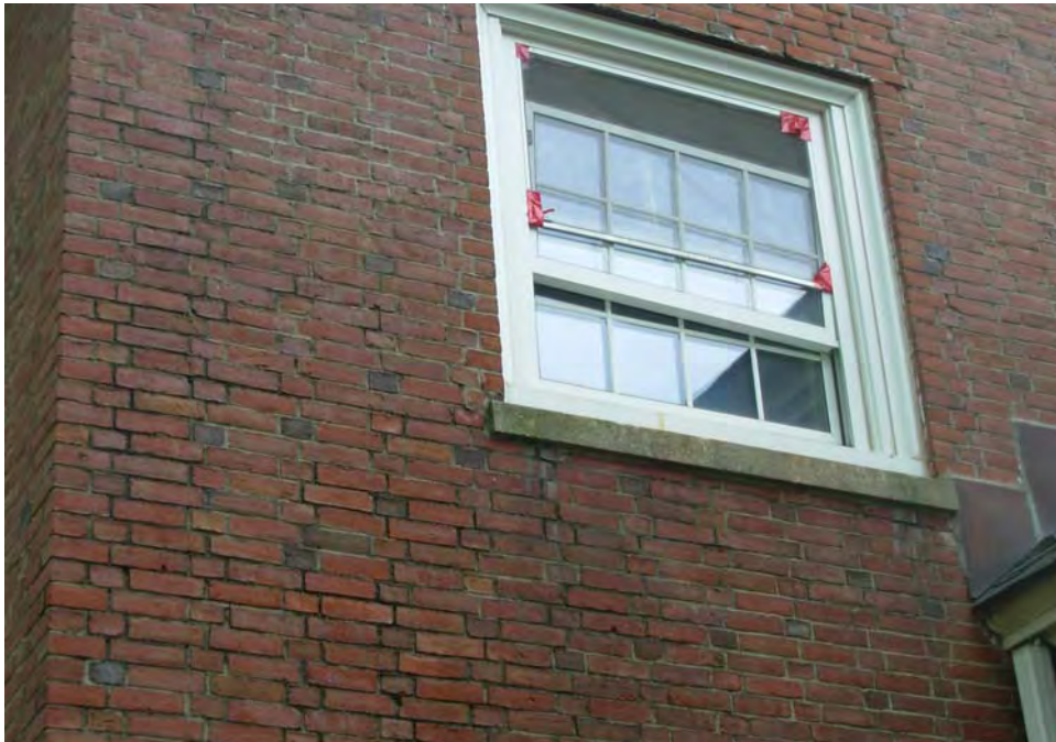
3. Mortar deterioration at some areas, to address
