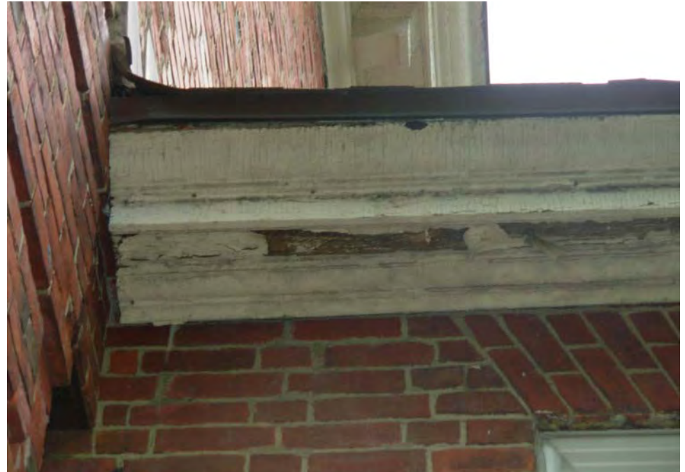
6. Wood trim and soffit deterioration
